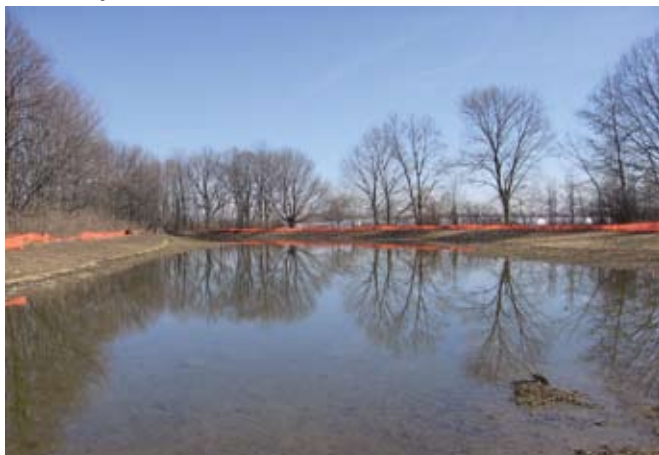
Clover-Groff ditch was reconstructed using an “over-wide” ditch design (left); less than one year later it already offers ecological benefits.
