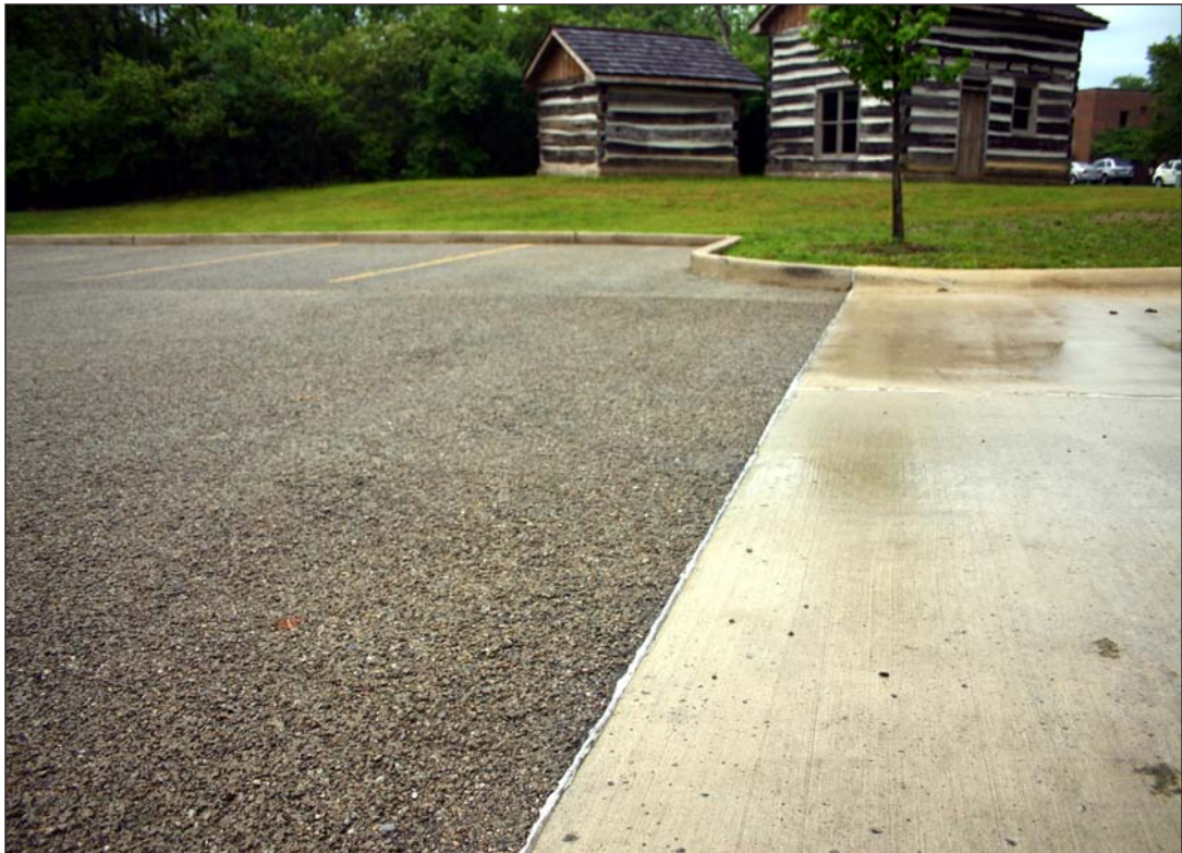
Figure 2.11.1 Porous Concrete at Indian Run Park in Dublin, Ohio.
