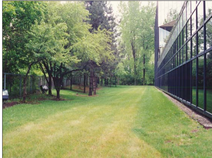
Figure 2.11.8 Vegetated Grid System utilized for fire access.
