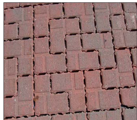
Figure 2.11.7 Pervious Interlocking Concrete Pavement
