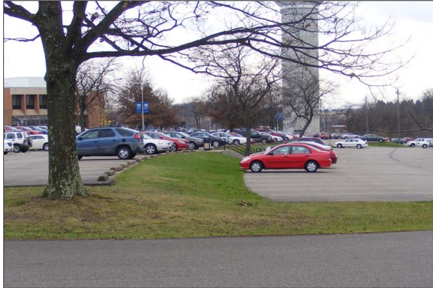
Figure 2.11.3 Terrace sloping areas to limit the pavement slope (photo credit: Brandon Andreson).
